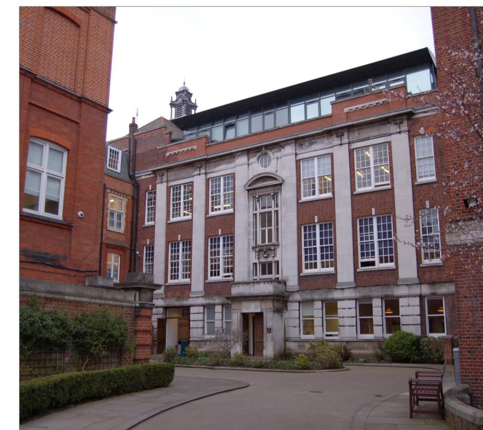
Stonework is used for the School buildings in the Science Block Quad
