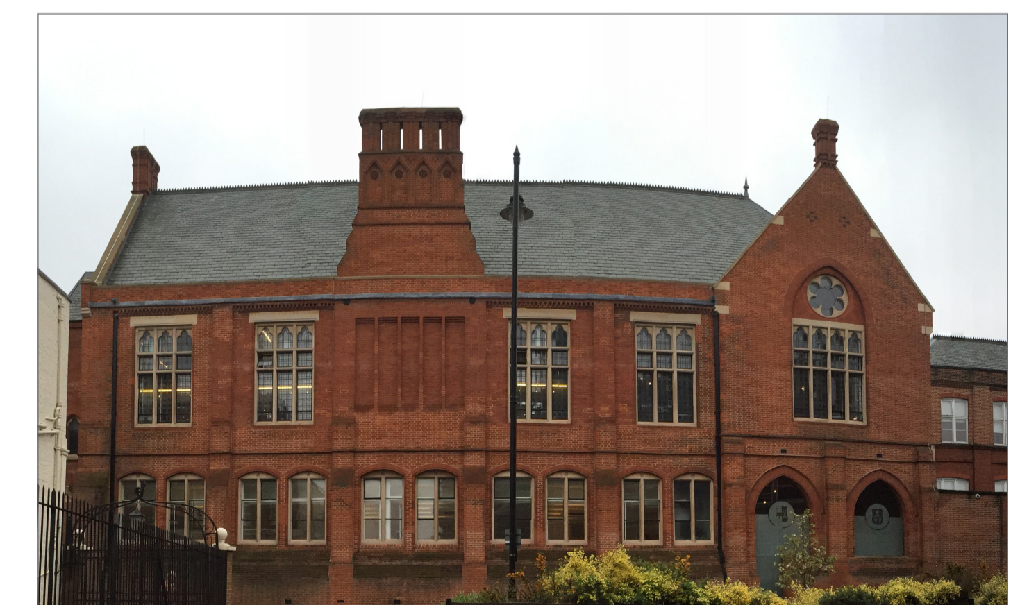
The Big School directly opposite Dyne House has a vertical emphasis to its fenestration
