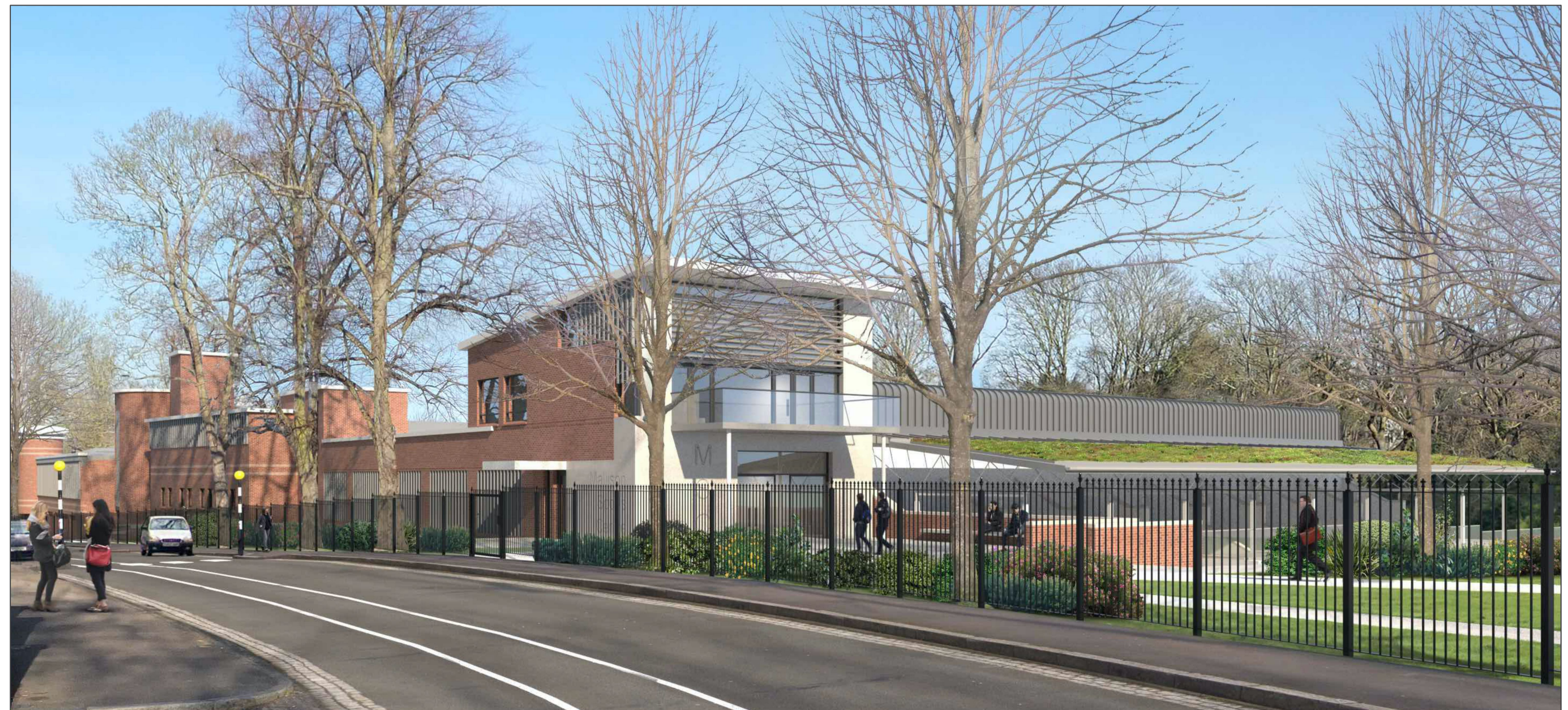
CGI perspective - view of project from south looking at main entrance and Fives court roof [to right]
